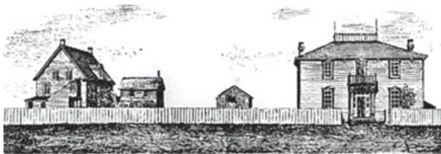
In Winnipeg, in 1880, construction began on a new St. Mary's church, which later became St. Mary's Cathedral. It was blessed in September 1881 and solemnly consecrated by the Archbishop of Montreal on September 25, 1887. Land was also acquired for St. Mary's Cemetery in the Fort Rouge area of the city.
